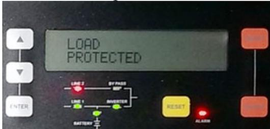
*Fig. 6. The indication of the power module with a built-in static bypass indicates that the power module is working in on-line mode, but bypass line is not available.*
